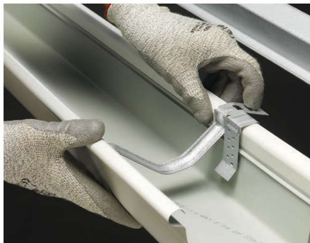
Step 3: Attaching the gutter overstrap
