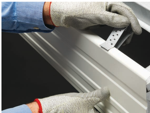
Step 1: Preparing to attach spring clip
